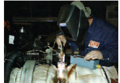
Narrow Groove Welding
